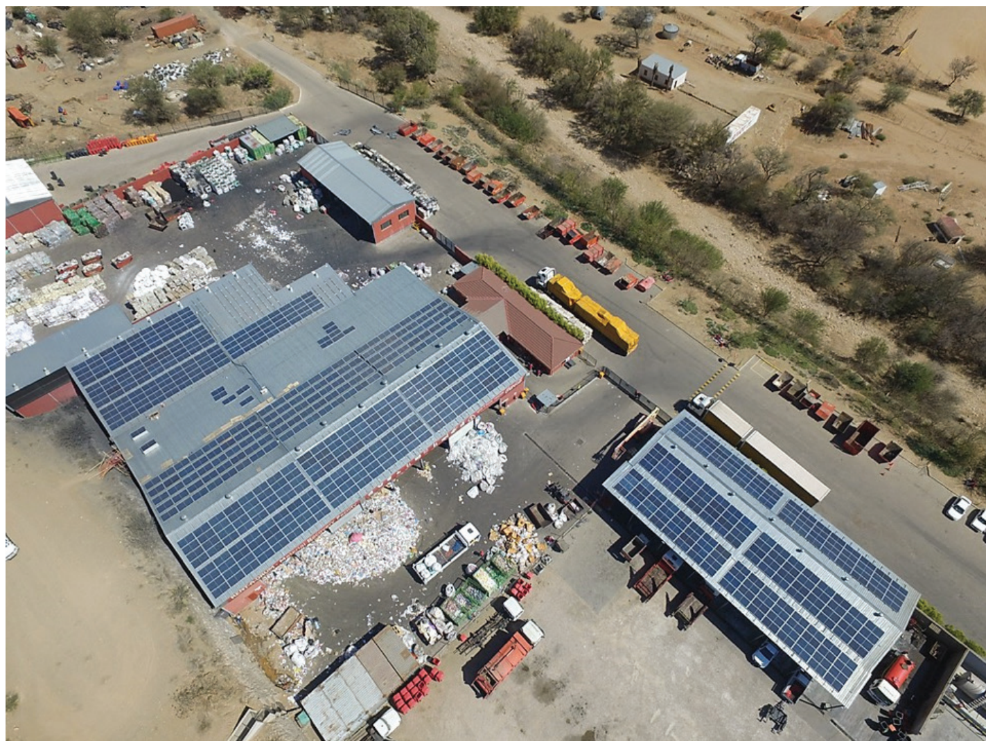
Figure 9: Installation of Project S-PV 5
