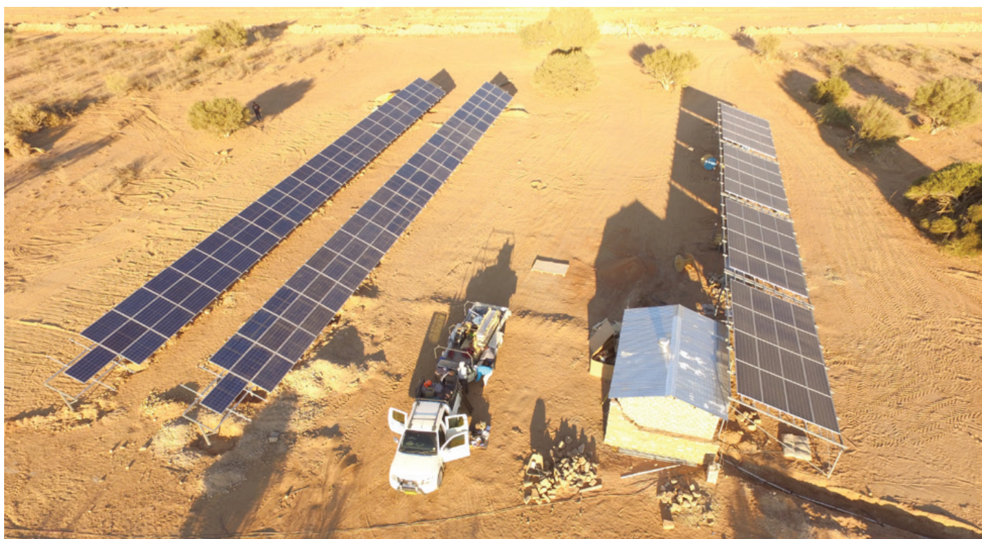
Figure 5: Installation of Project S-PV 1
