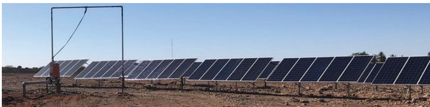
Figure 6.2: Installation of Project S-PV 2
