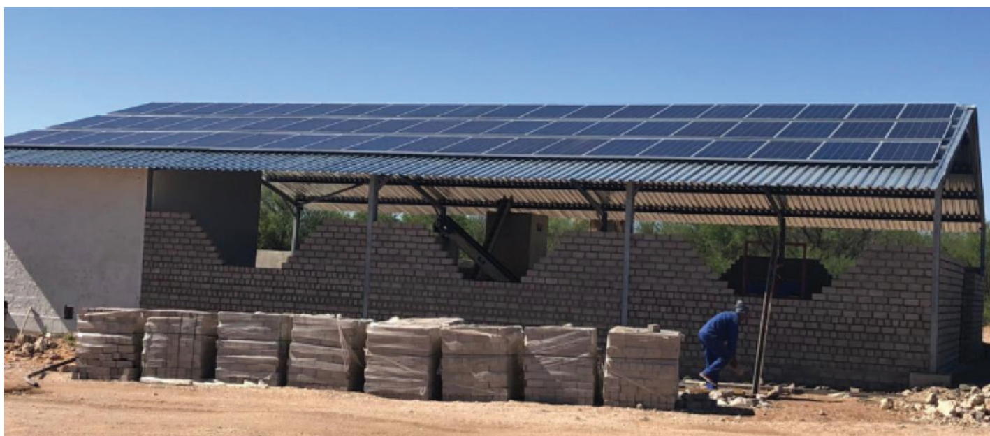
Figure 6.1: Installation of Project S-PV 2
