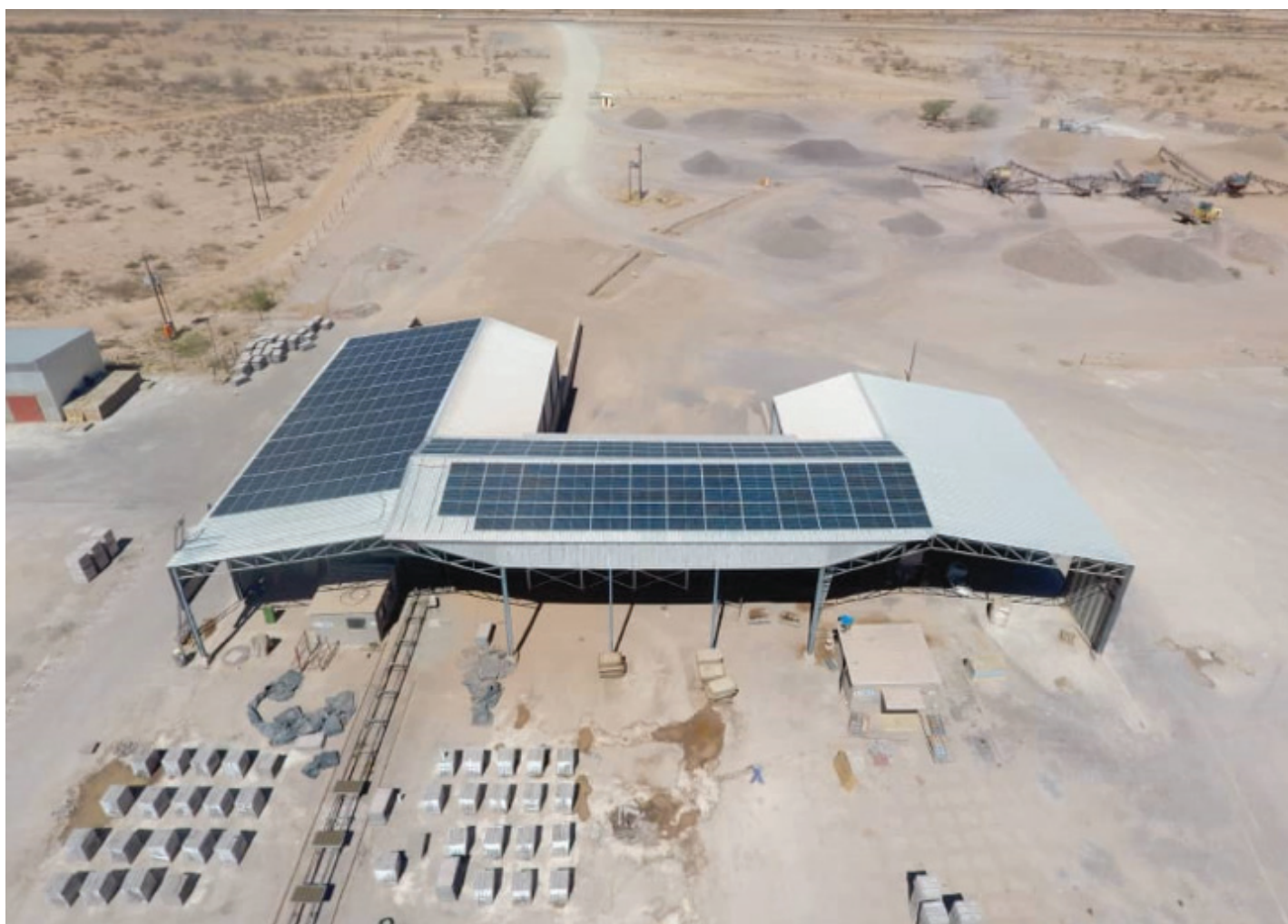
Figure 8: Installation of Project S-PV 4 (Mariental)
